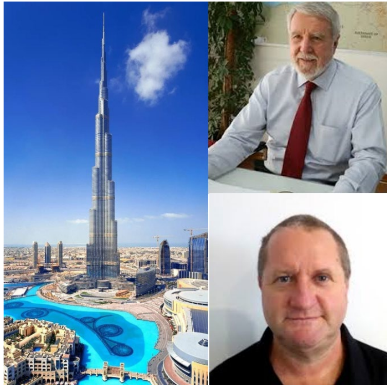
Figure 16: Architect drawing of Burj Khalifa, Dubai (left), Ian Sparks, surveyor of Petronas Tower A & Burj Khalifa (above right) and Rob Fulloon, surveyor of Petronas Tower B (below right).
