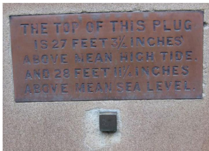
Figure 1: Survey plug (now PM50000) on the external northern wall of the former Department of Lands building in Bridge Street, Sydney.
