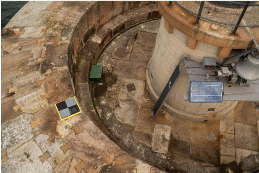
Figure 5: A Propeller Aeropoint ground control point in place at the capture site.
