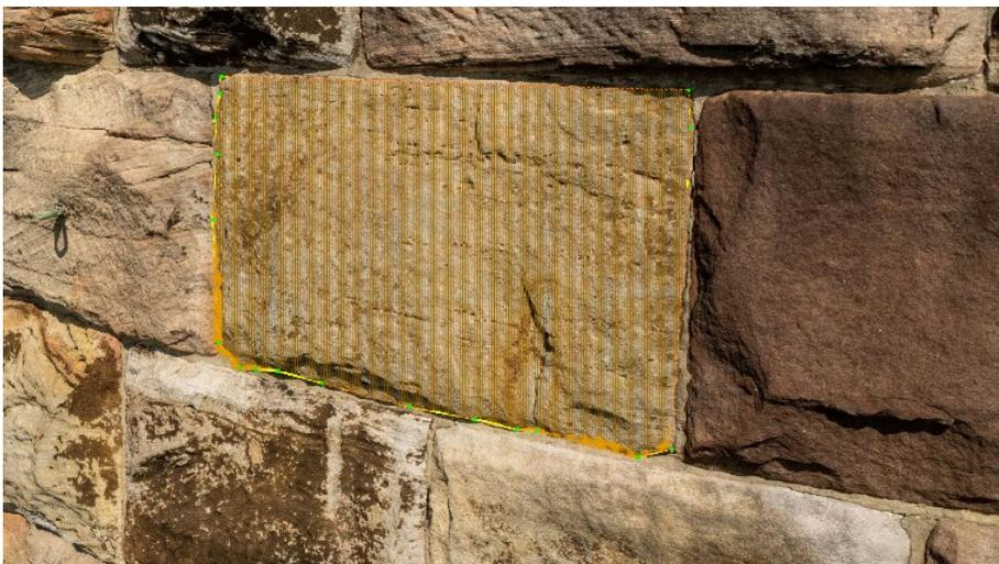
Figure 24: Measurement capability within the 3D reality model for precise measurements of sandstone.
