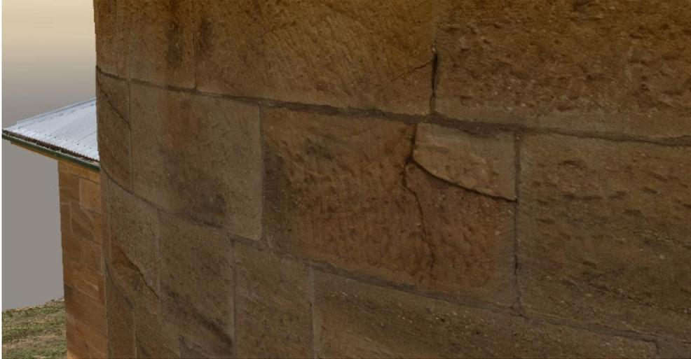
Figure 19: Level of detail, clearly showing cracks in Hartley Historic Courthouse 3D reality model.
