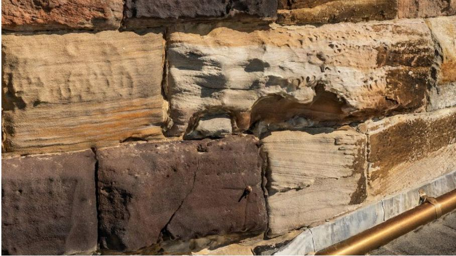
Figure 22: Level of detail, clearly showing cracks and weathering in Fort Denison 3D reality model.
