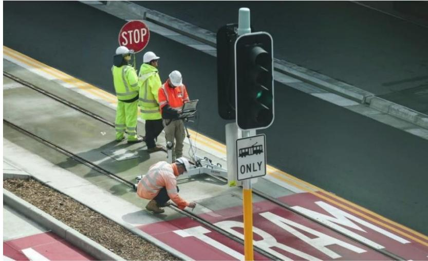
Figure 1: Monteath & Powys staff operating an Amberg rail trolley for conformance of the track prior to running the first light rail vehicle (image courtesy of Newcastle Herald).
