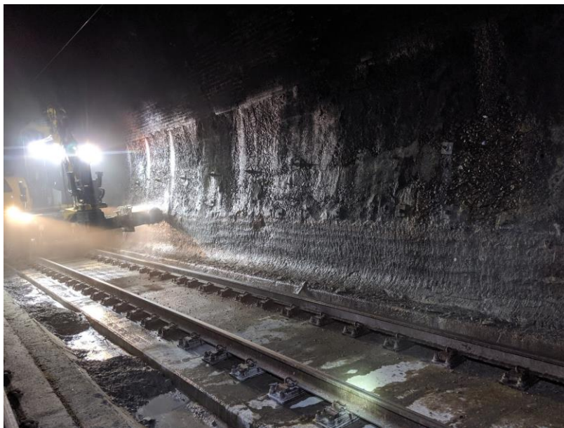
Figure 3: Tunnel Trimmer in use.
