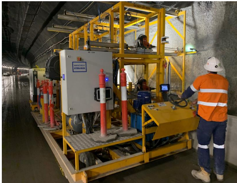
Figure 2: Paneller in use (NorthConnex tunnels).
