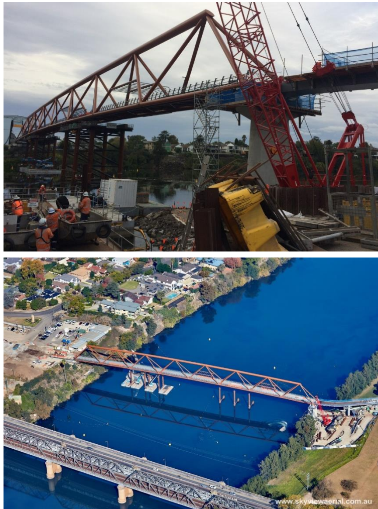
Figure 20: Construction of the Nepean River Green Bridge.
