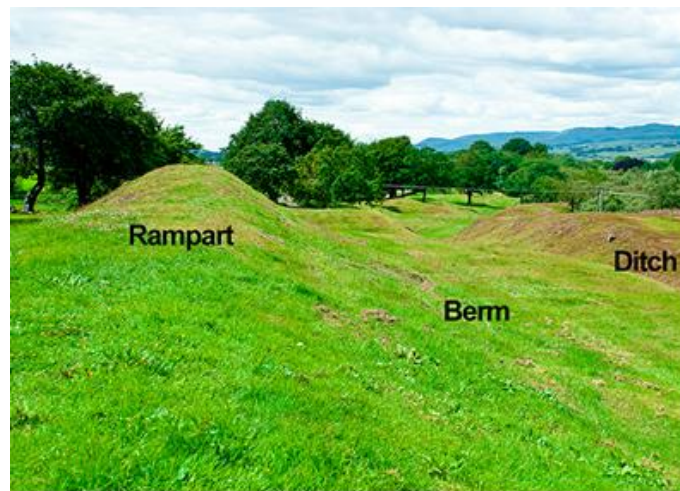
Figure 2: Typical view of the design of the Antonine Wall, showing the rampart, berm and ditch as it crosses the countryside.
