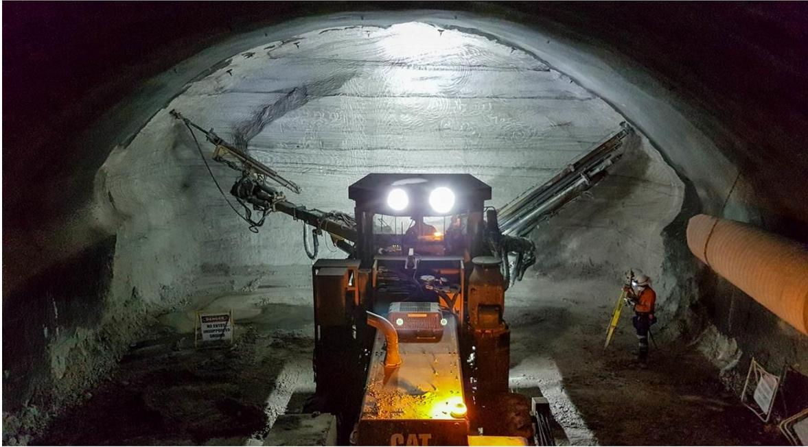
Figure 1: Bolting, grouting, survey as-builts and convergence monitoring in close proximity.
