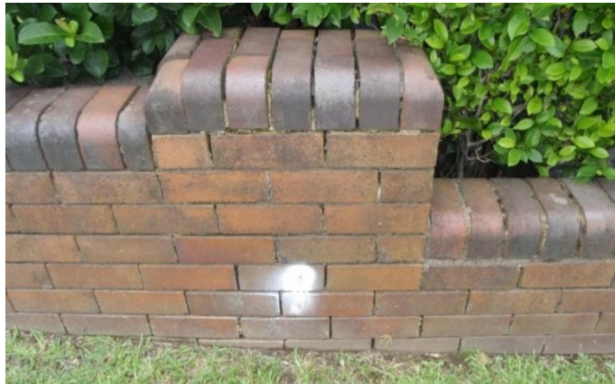
Figure 15: 'Roof nail and cut' in old brick fence in DP419960 (1959), placed after Eltham Street was re-established using a pair of found stone alignment posts.
