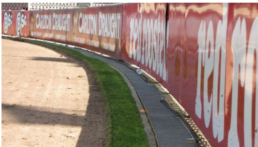
Figure 4: concrete edge drain.
