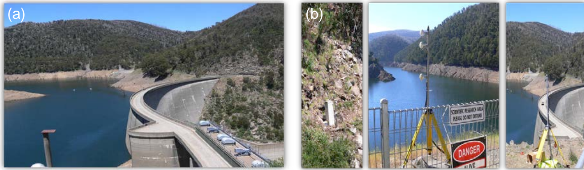
Figure 4: (a) Tumut Pond Dam (total view), and (b) LocataLite and receiver installation.
