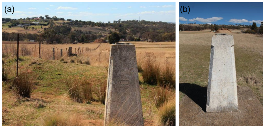
Figure 3: (a) Pillar 2 looking north (note contour bank added after construction), and (b) Pillar 4 looking south (note council gravel stockpile on line).
