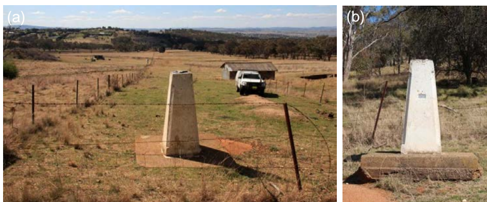
Figure 1: (a) Pillar 1 looking north along Bathurst baseline (note rifle range to the east), and (b) Pillar 1 looking south (note effects of erosion).
