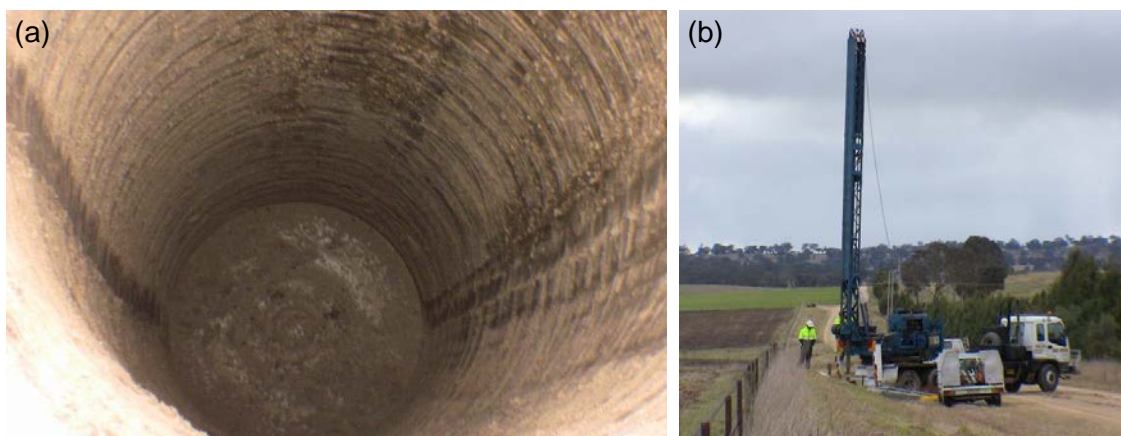
Figure 10: (a) Typical finished borehole, and (b) boring machine at Pillar 3.
