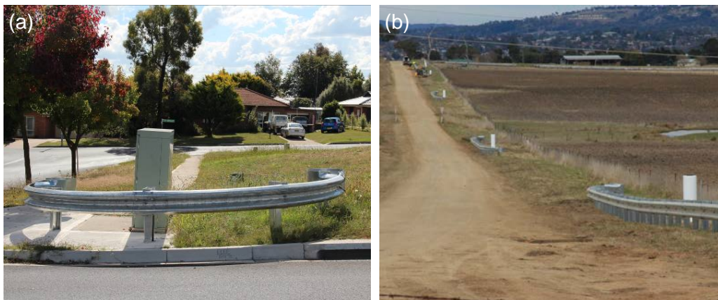
Figure 15: (a) Safety barrier type initially deemed adequate, and (b) final safety barrier installation.
